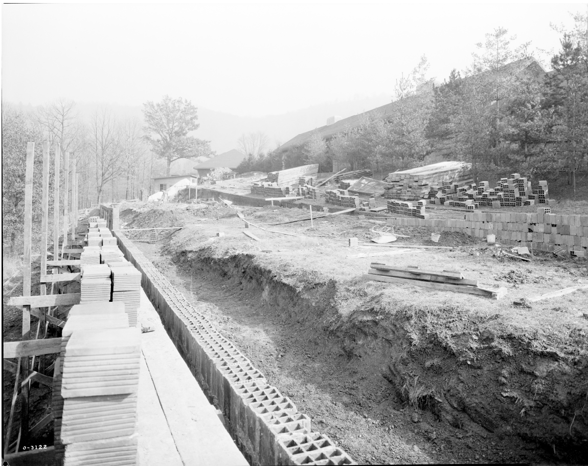
1929. Tile block wall construction on lower side of Biltmore Industries dye vat building
